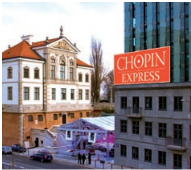
Warszawa, Tamka 43: nasza siedziba | 43 Tamka Street, Warsaw: our headquarters
